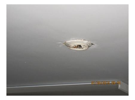
Smoke detector where leakage came through.
