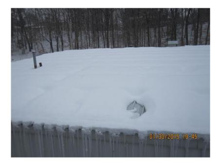
Melted snow above insulation gap.
